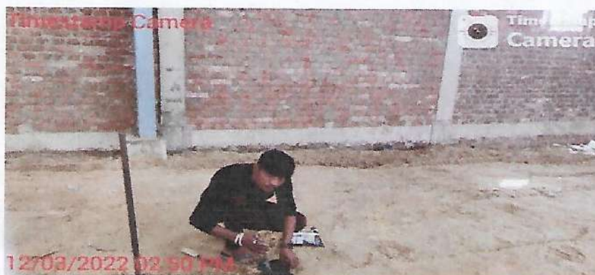
CORE CUTTER TEST ON SITE FOR DENSITY
