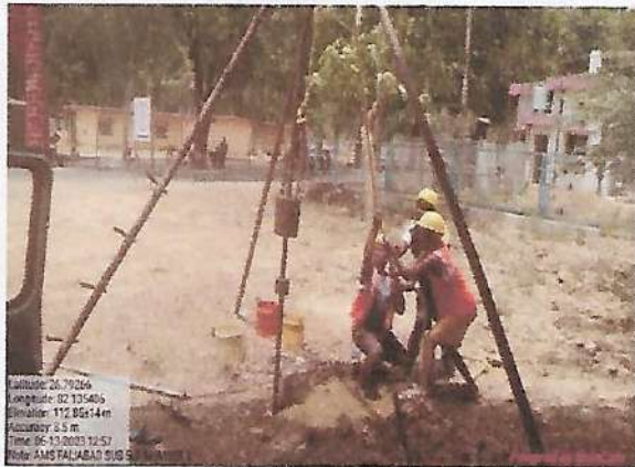
S.P.T TEST ON SITE FOR FOUNDATION
